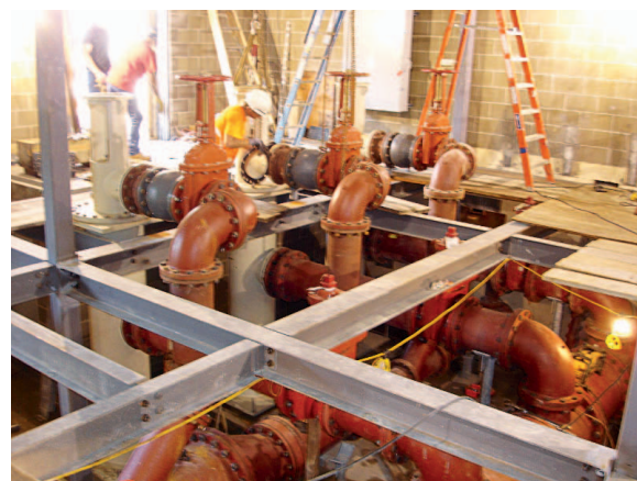
Quaker Lane transmission pump station rehabilitation project.
