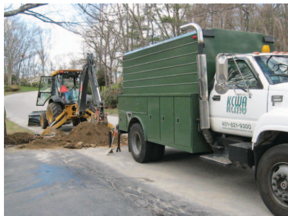
Water main repair.
