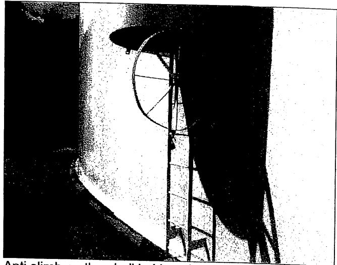
Anti climb on the shell ladder with a lock
