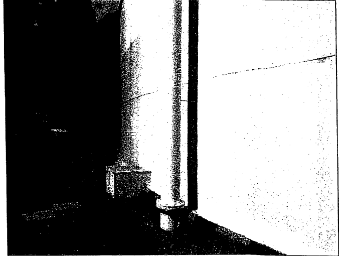
Overflow pipe enters into the ground
